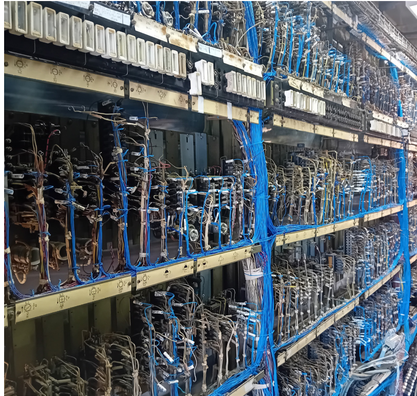
“Old” relay frames with their – several times modified - wiring
