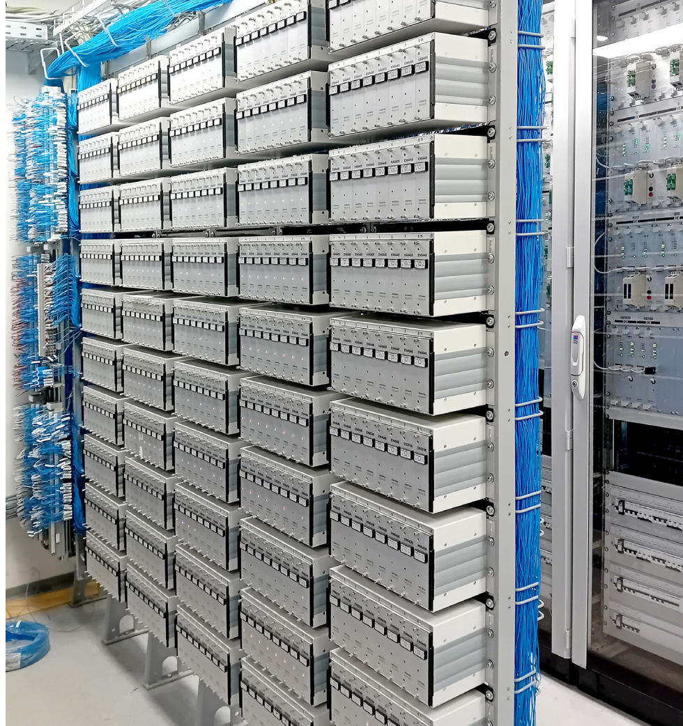
Relay frames with adaptation relays, PRORIS-H in background
