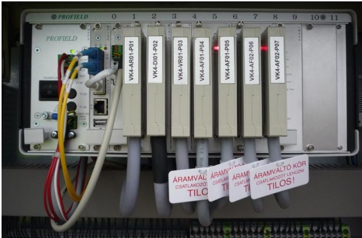
The intelligent controller of the system is the Prolan Profield RTU. It's configuration is more or less the same in every installation, only the current sensing circuitry may vary depending on the number of the connected turn-outs.
