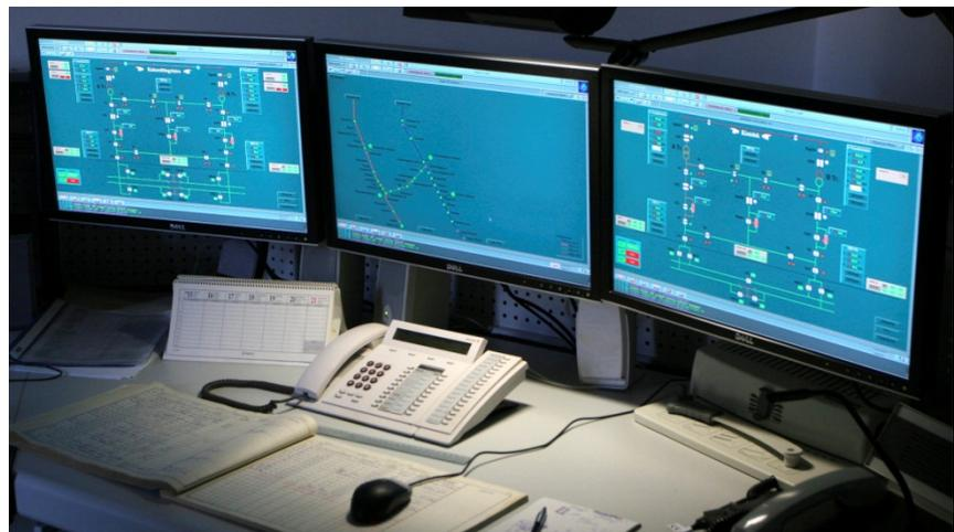
The display shows the schematic layout of the station and all the relevant data related to the heating status. The example below is the monitor screen of a Hungarian middle sized station:
